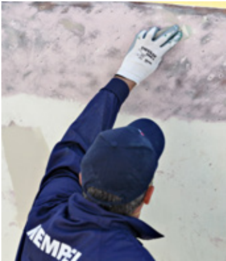
Fill along boottop
