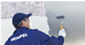
Apply Hempel's Underwater Primer onto prepared surface
