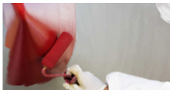
Applying antifouling
