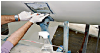
Wet scrape to remove old antifouling
