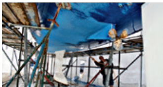
Clean abraded surface
