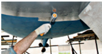
Apply Hempel's High Protect with roller
