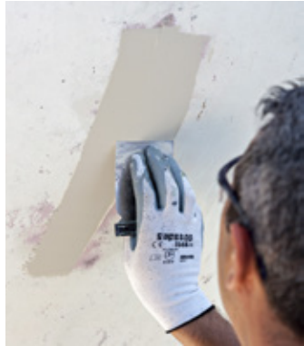
Fairing any defects
